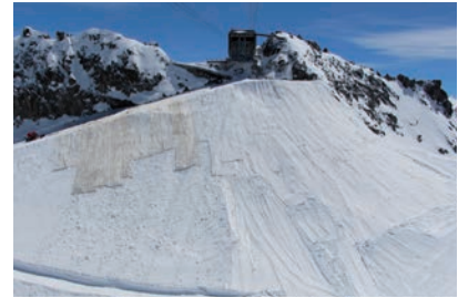
Fleece to prevent ice loss on the access ramp.
