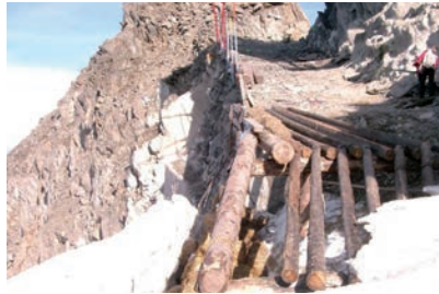
Ramp construction to enable skiers to access slopes on the glacier.
