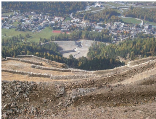
High costs for a protection dam against debris flows due to permafrost melting, Pontresina, Switzerland.
